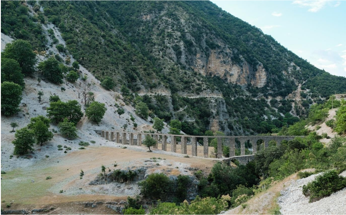
Figure 2: 19 th -century aqueduct over the Bënça River, a tributary of Vjosa
