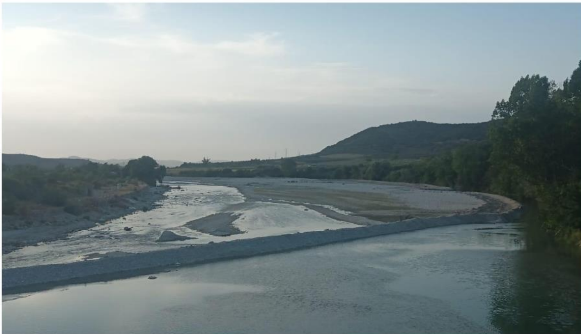
Figure 10: Irrigation channels on the Shushica River branch (Picture: NAPA)
